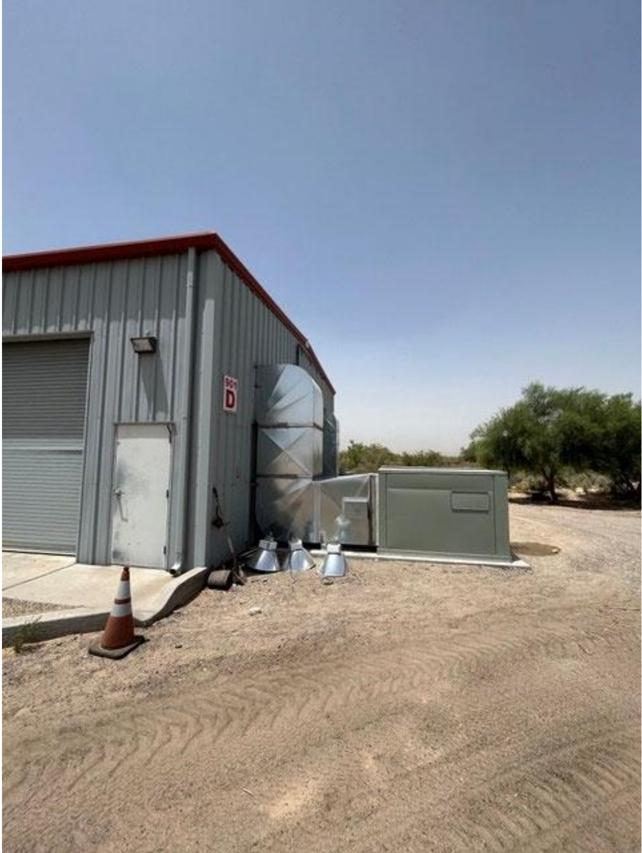
PHOTO OF NORTH SIDE OF BUILDING
