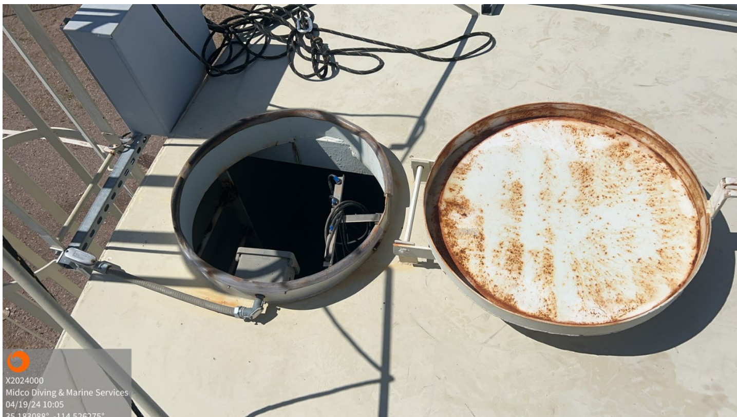
Access Hatch – Coating Failure with Corrosion Noted
