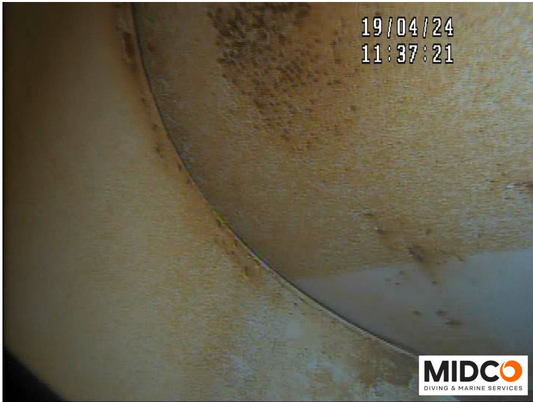
Man Entry #2 – Coating Failure with Corrosion Noted
