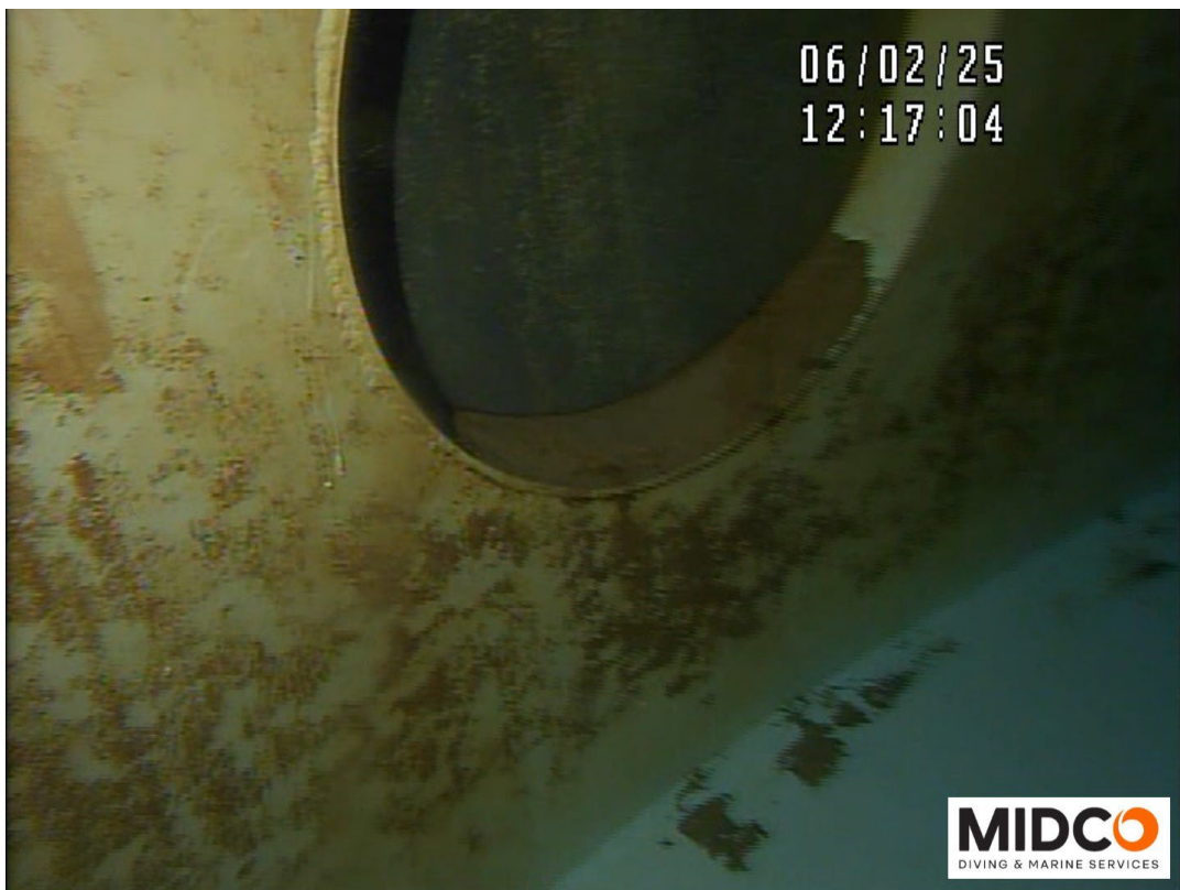
Man Entry #2 – Coating Failure with Corrosion Noted
