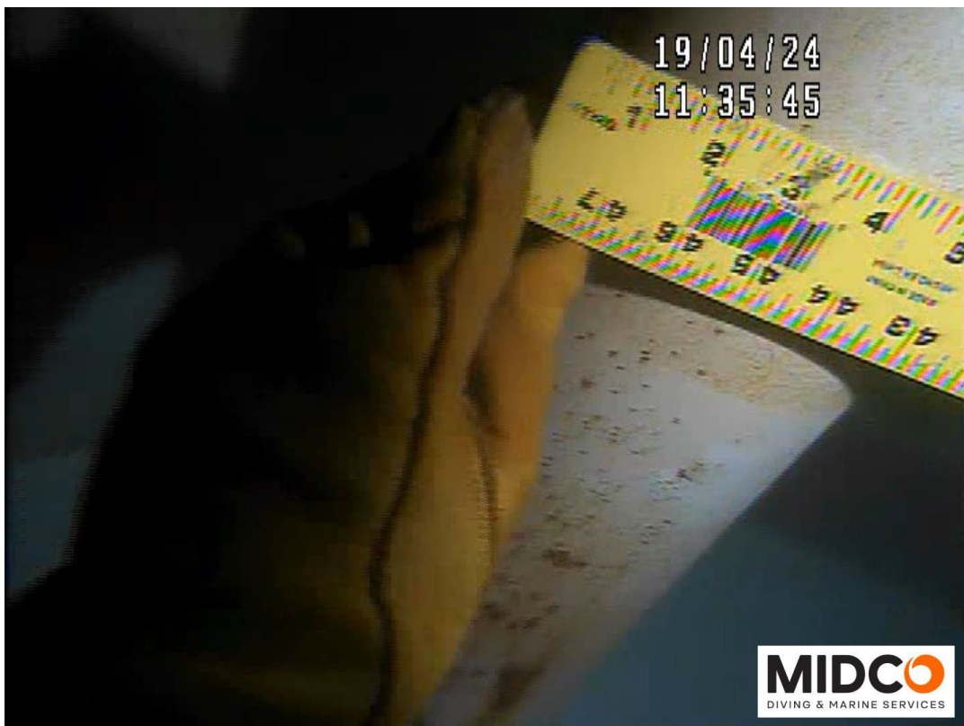
Overflow Plumbing – Coating Failure with Corrosion Noted
