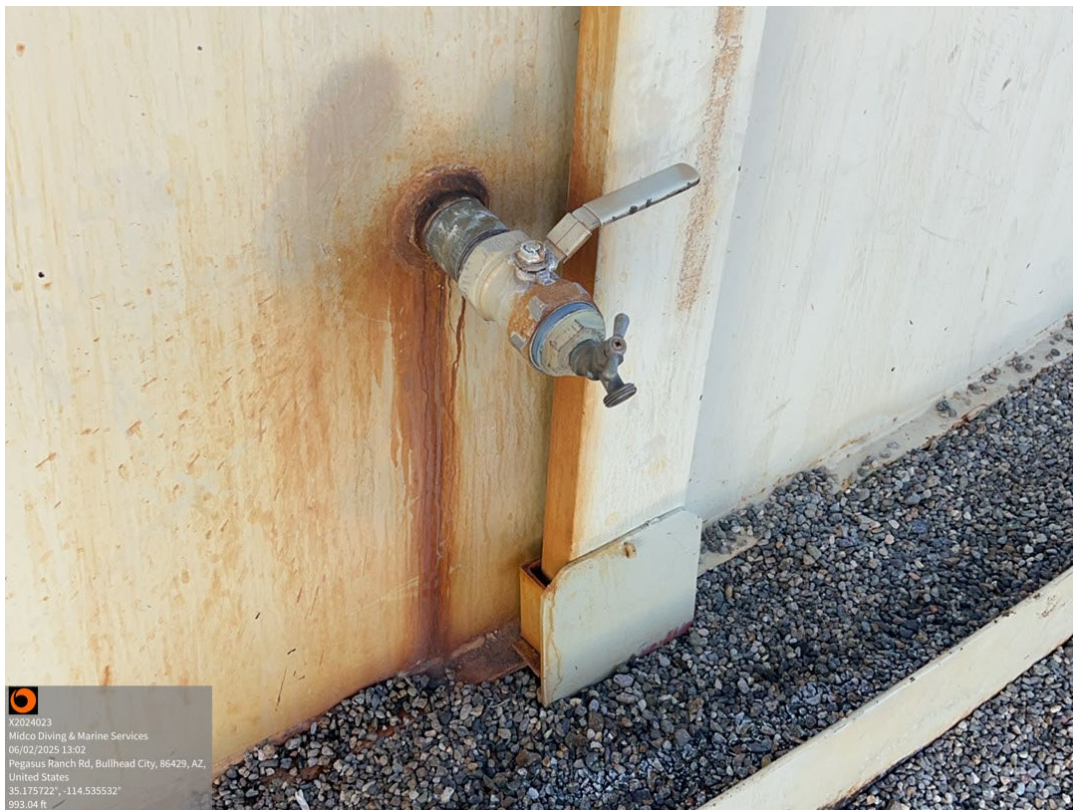
Water Tap & Manual Level Indicator – Non-Functioning
