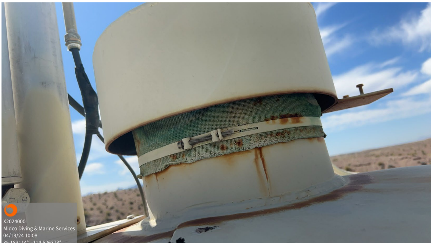
Roof Vent Screen – Not #24 Mesh
