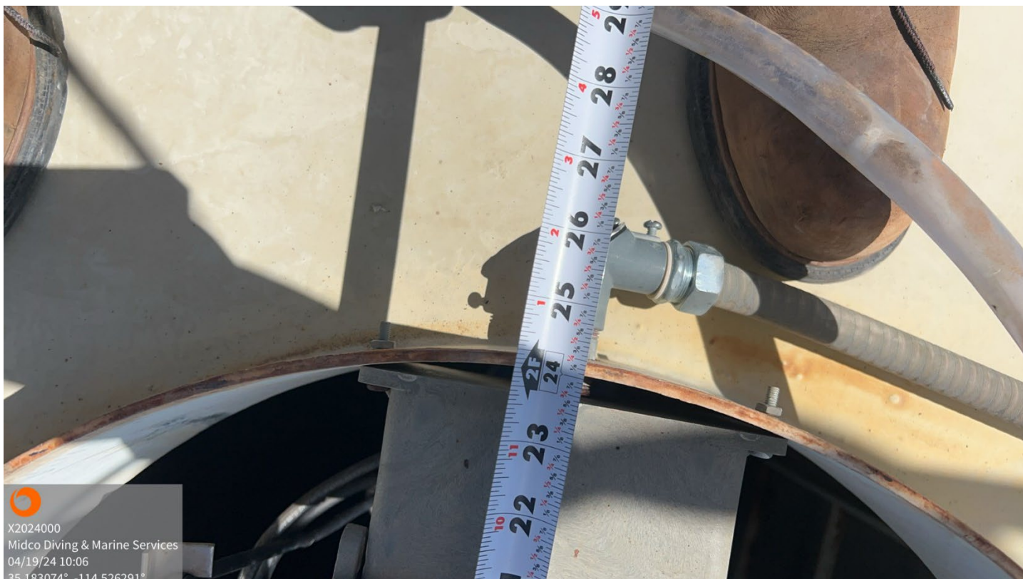
Access Hatch – Coating Failure with Corrosion Noted
