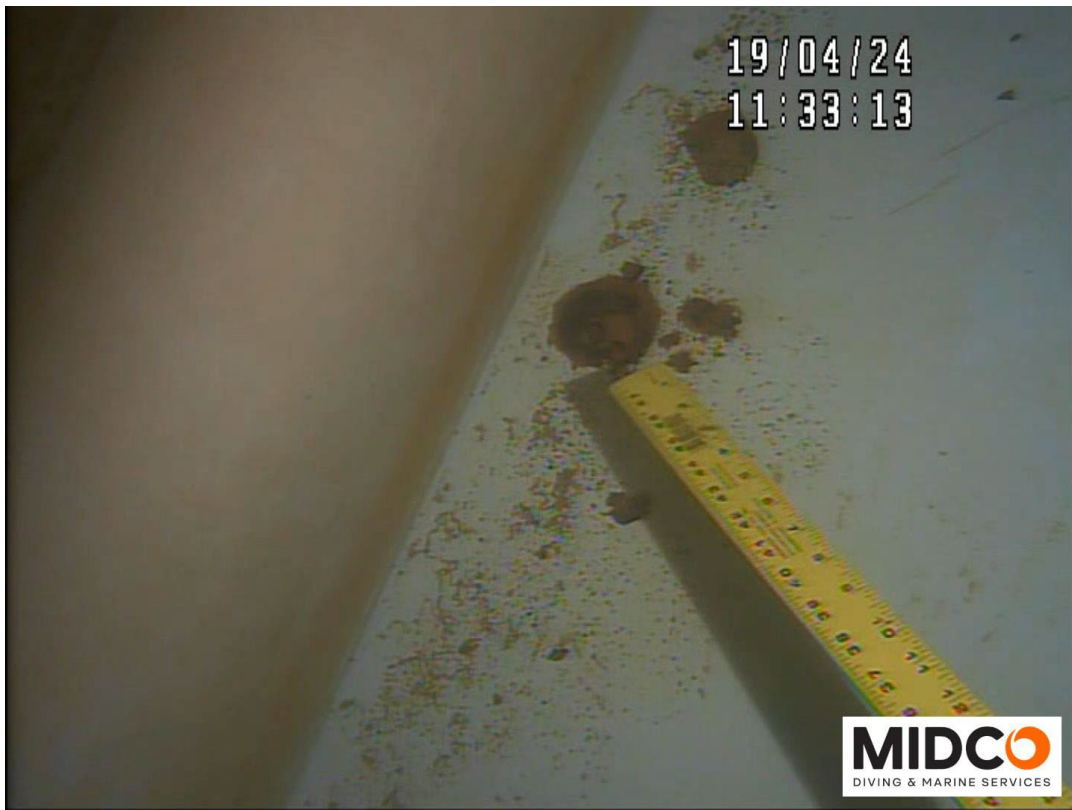
Typical Floor – Coating Failure with Corrosion & Pitting Noted
