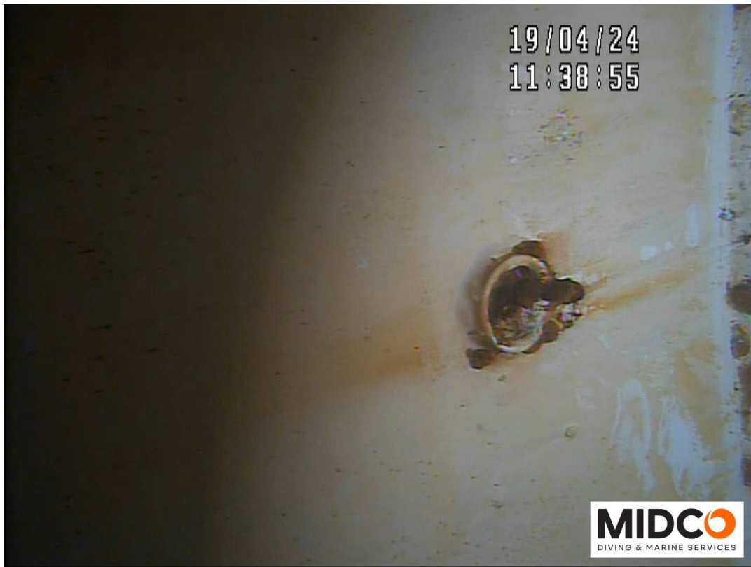
Interior Water Tap – Coating Failure with Corrosion Noted
