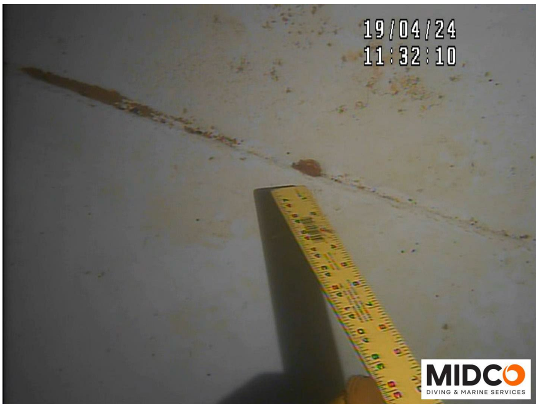
Typical Floor – Coating Failure with Corrosion Noted
