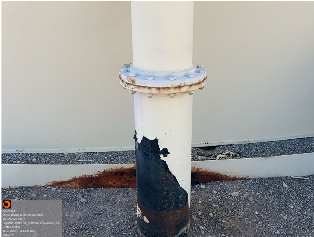
Overflow Plumbing – Coating Failure with Corrosion Noted
