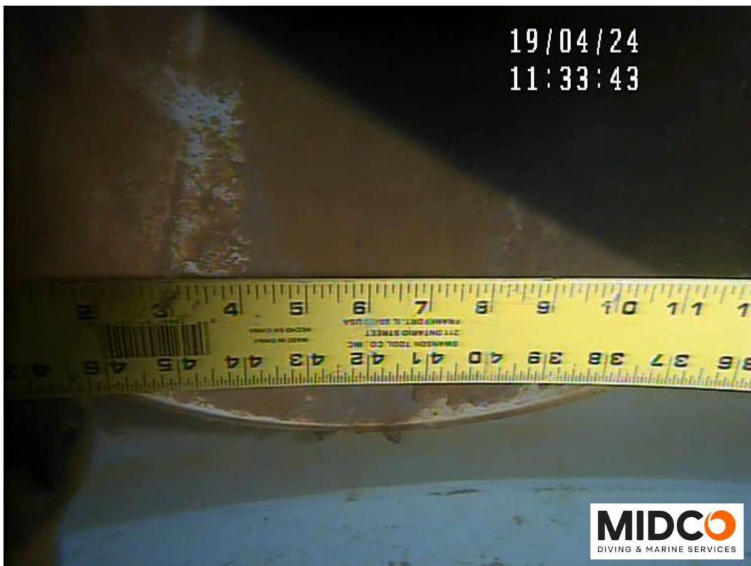
Inlet Plumbing – Coating Failure with Corrosion Noted
