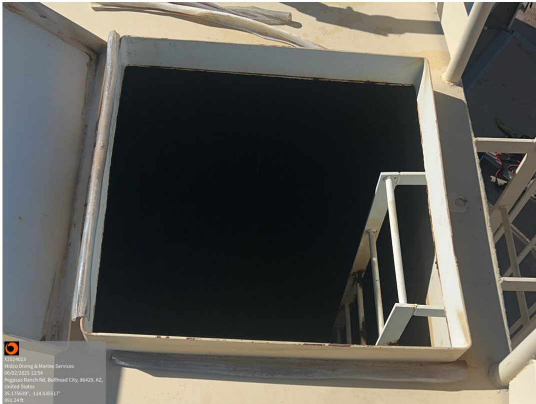
Access Hatch – Weather Stripping Deterioration Noted
