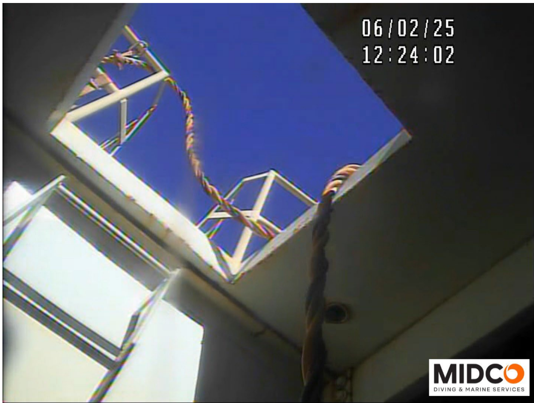
Access Hatch – Coating Failure with Corrosion Noted
