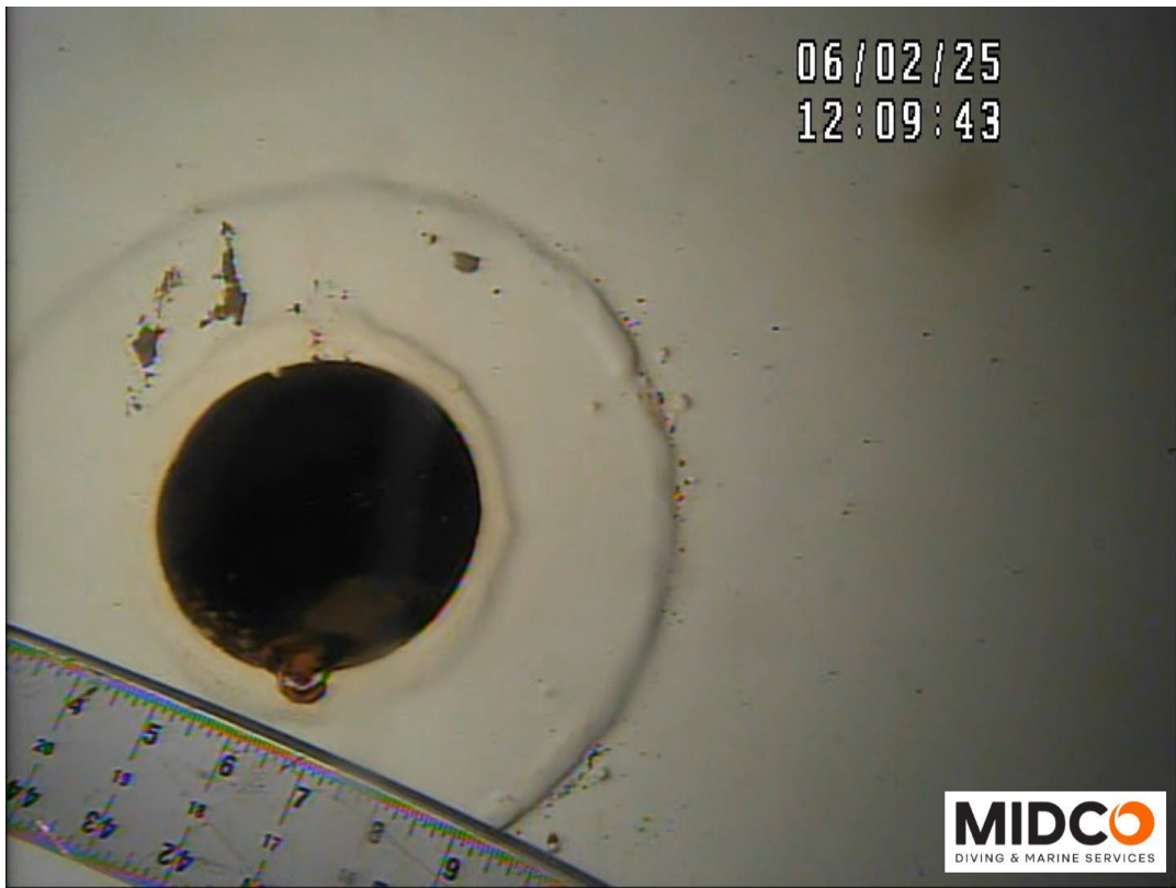
Drain Plumbing – Coating Failure with Corrosion Noted
