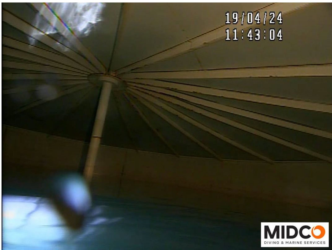
Typical Roof & Rafters – Coating Failure with Corrosion Noted
