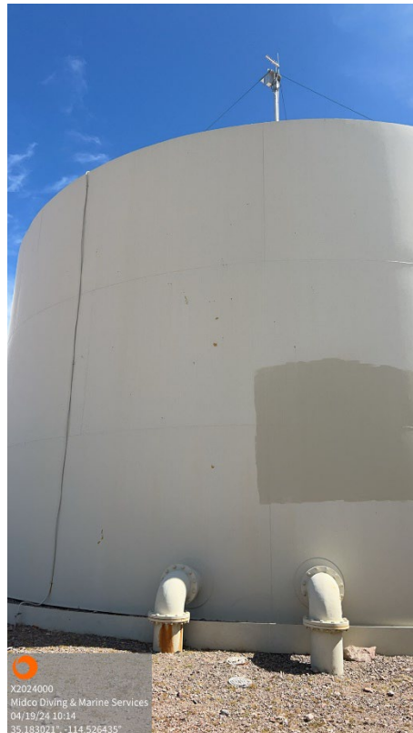
Exterior Reservoir – Coating Failure; Previous Repairs Noted
