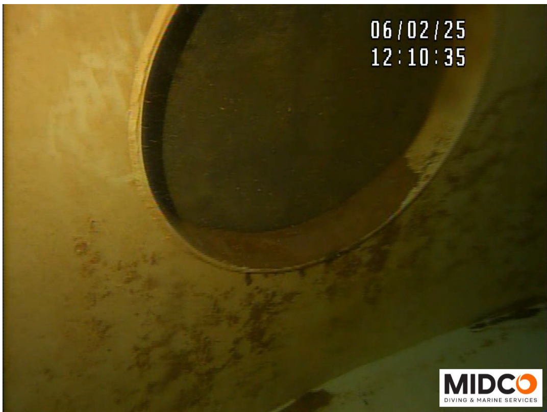
Man Entry #1 – Coating Failure with Corrosion Noted
