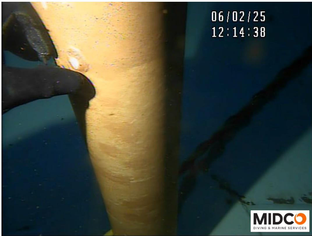
Center Column – Coating Failure Noted
