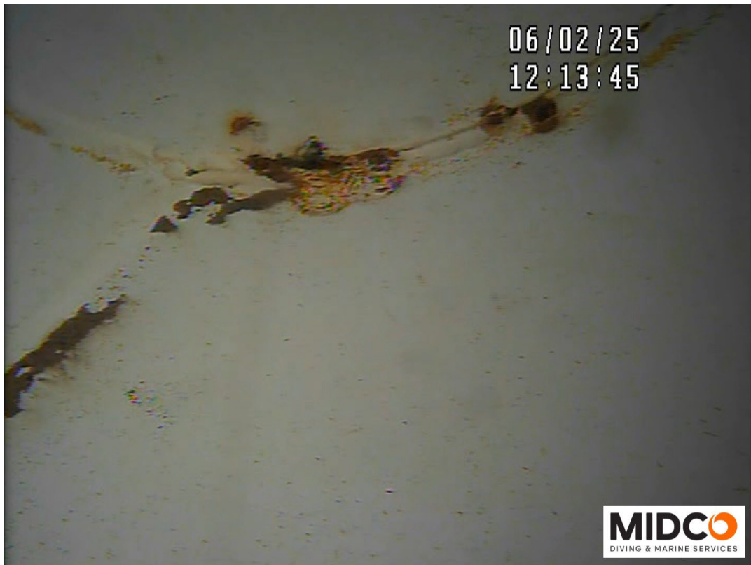
Center Column Base – Coating Failure with Corrosion Noted
