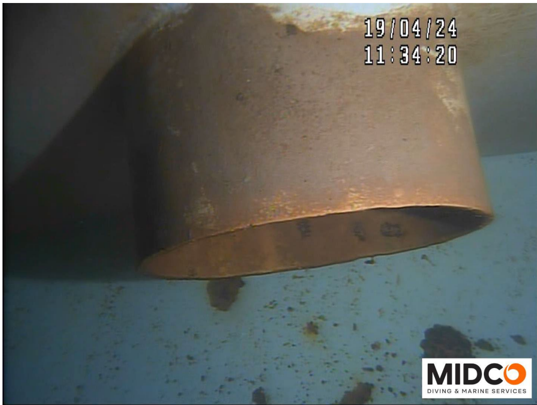
Outlet Plumbing – Coating Failure with Corrosion Noted
