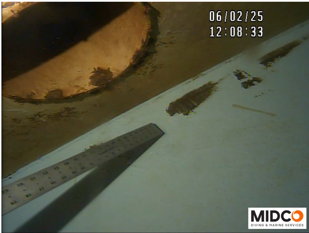
Inlet Plumbing – Coating Failure with Corrosion Noted
