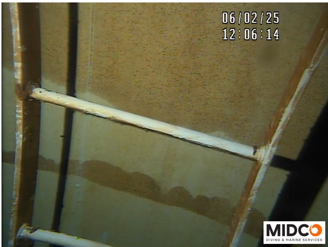
Interior Ladder – Coating Failure with Corrosion Noted
