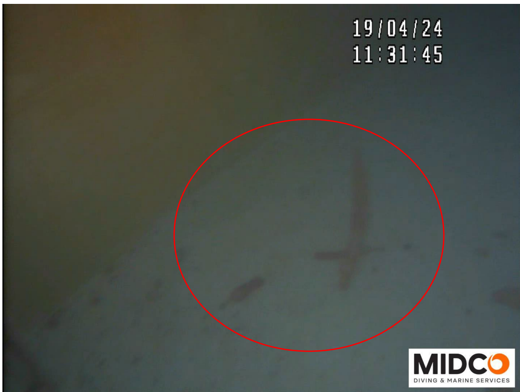
Cleaning Reservoir – Light Skiff of Sediment with Debris Noted
