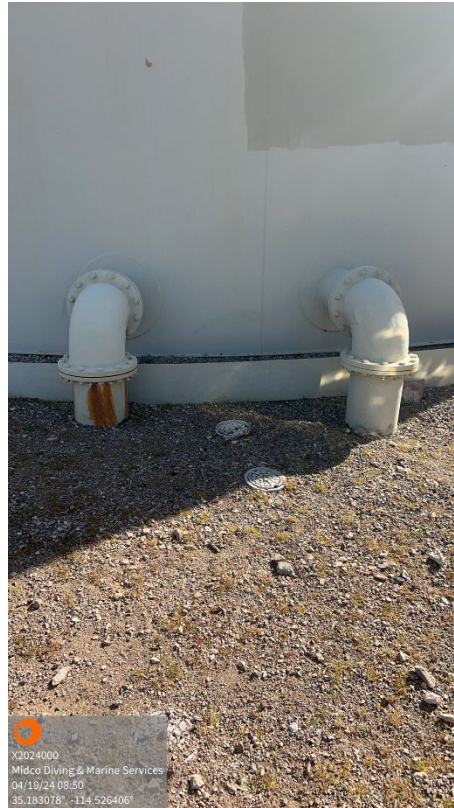
Inlet & Outlet Plumbing – Coating Failure with Corrosion Noted
