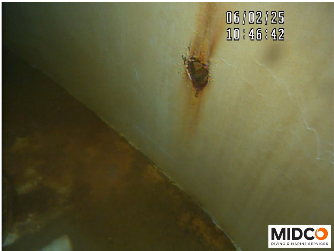
Water Tap – Coating Failure with Corrosion Noted
