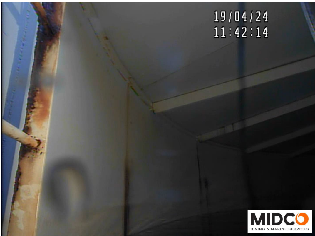
Wall to Roof Seam – Coating Failure with Corrosion Noted
