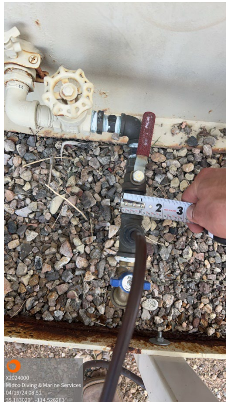
Exterior Water Tap – Coating Failure with Corrosion Noted
