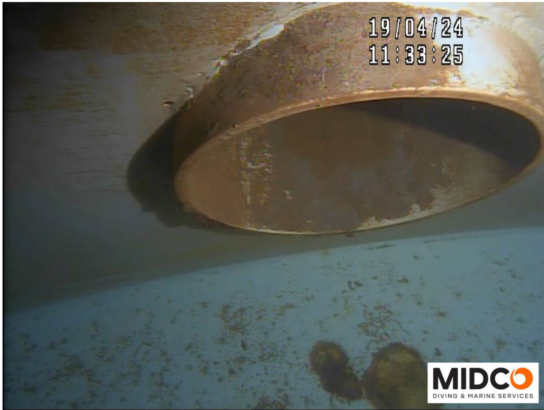
Inlet Plumbing – Coating Failure with Corrosion Noted
