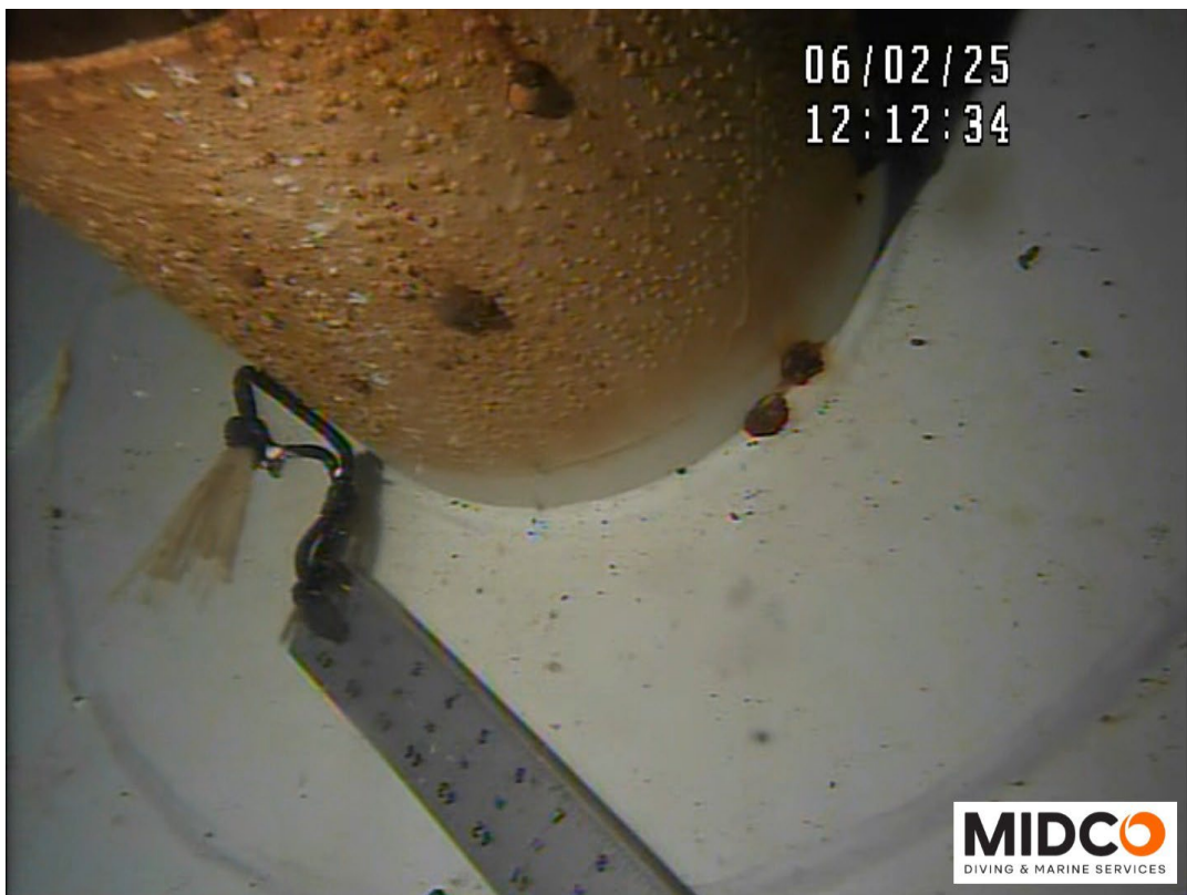
Outlet Plumbing – Coating Failure with Corrosion Noted
