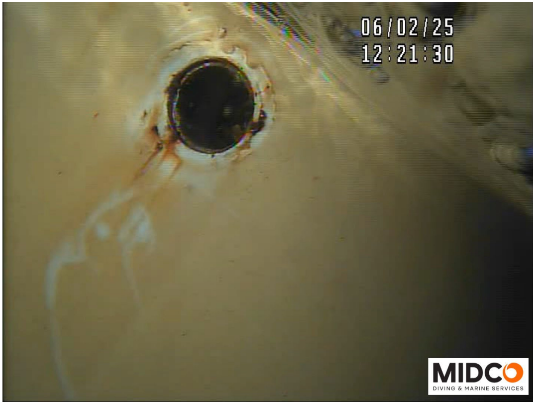
Interior Plumbing #1 – Coating Failure with Corrosion Noted
