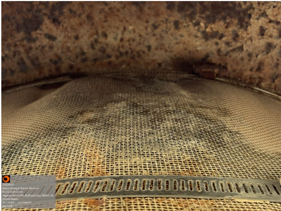
Roof Vent & Screen – Coating Failure with Corrosion Noted
