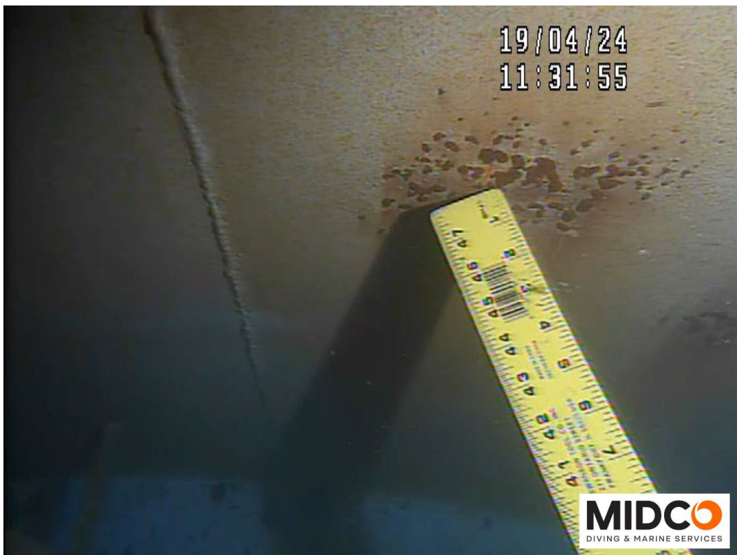
Typical Wall – Coating Failure with Corrosion Noted
