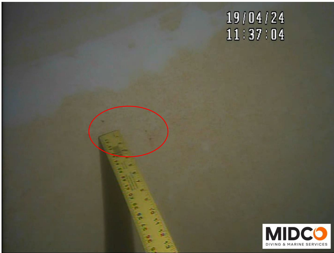
Typical Wall – Coating Failure with Corrosion Noted
