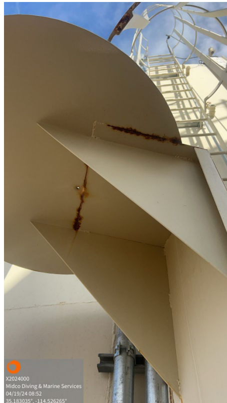
Exterior Ladder – Coating Failure with Corrosion Noted
