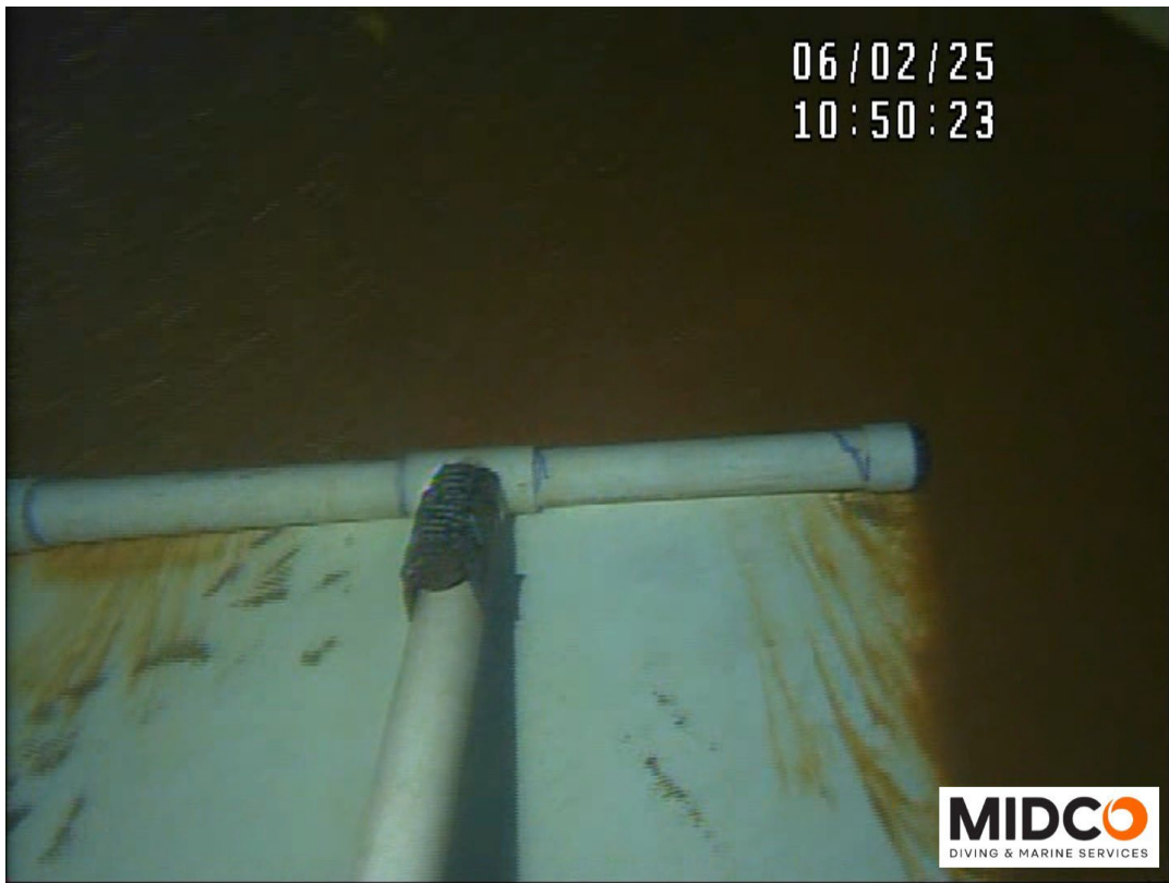
Cleaning Reservoir – Light Skiff of Sediment Noted
