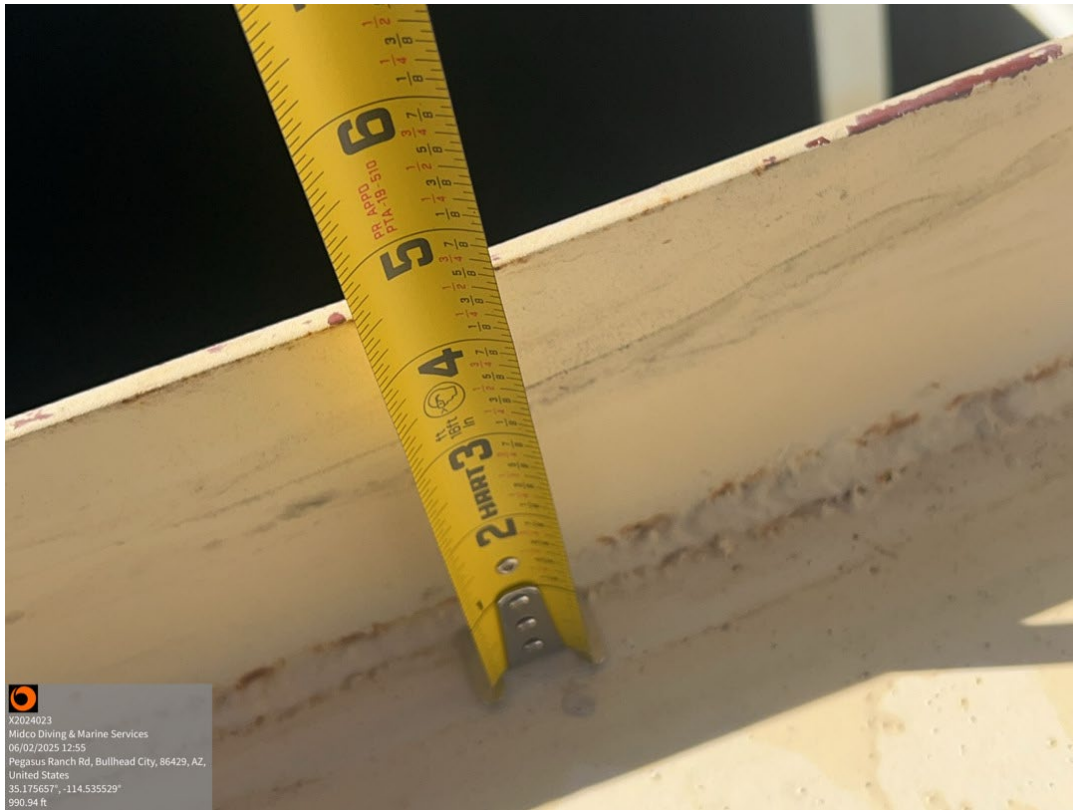
Access Hatch – Coating Failure with Corrosion Noted
