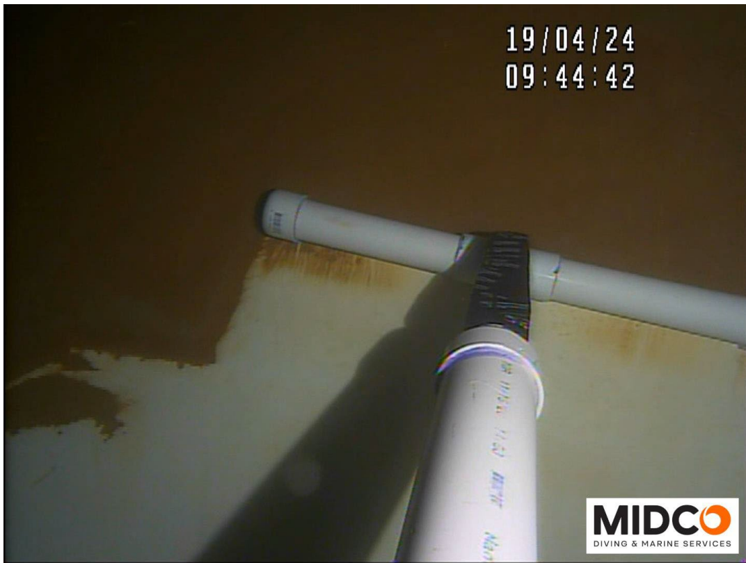
Cleaning Reservoir – Light Skiff of Sediment Noted
