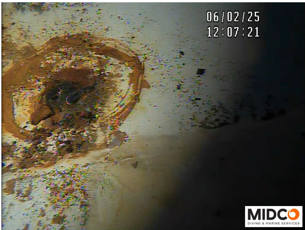
Manual Level Indicator – Floor Anchor Deterioration Noted
