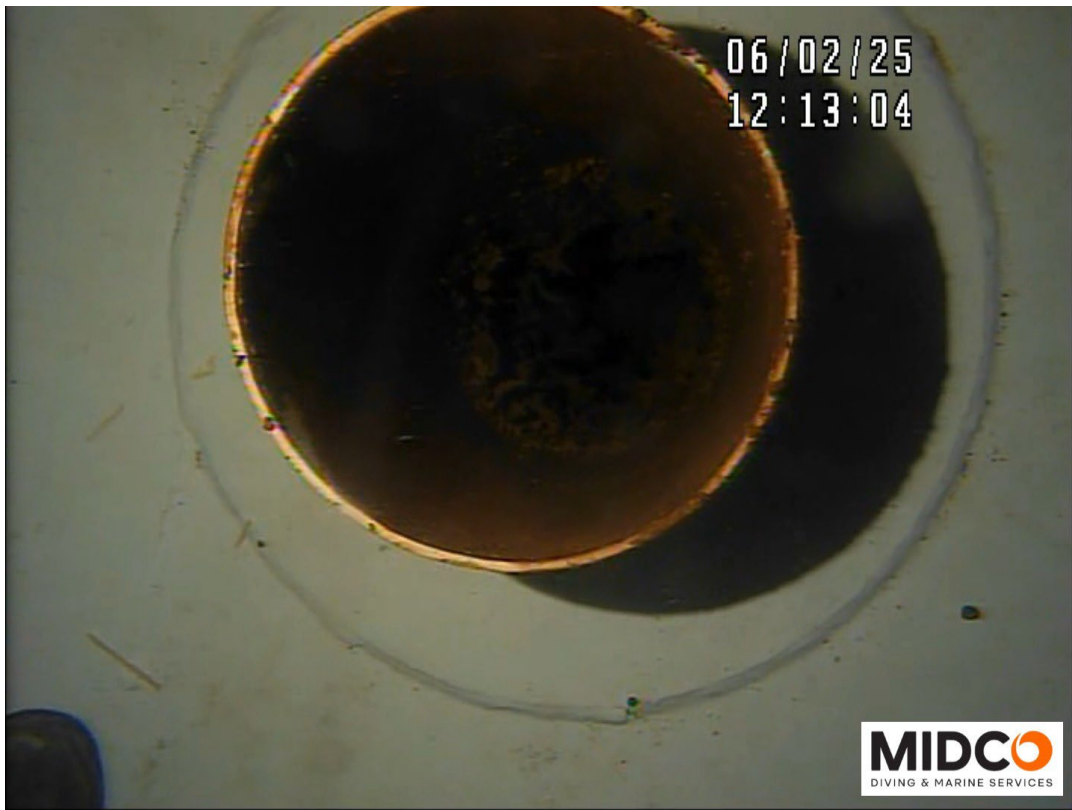
Outlet Plumbing – Coating Failure with Corrosion Noted
