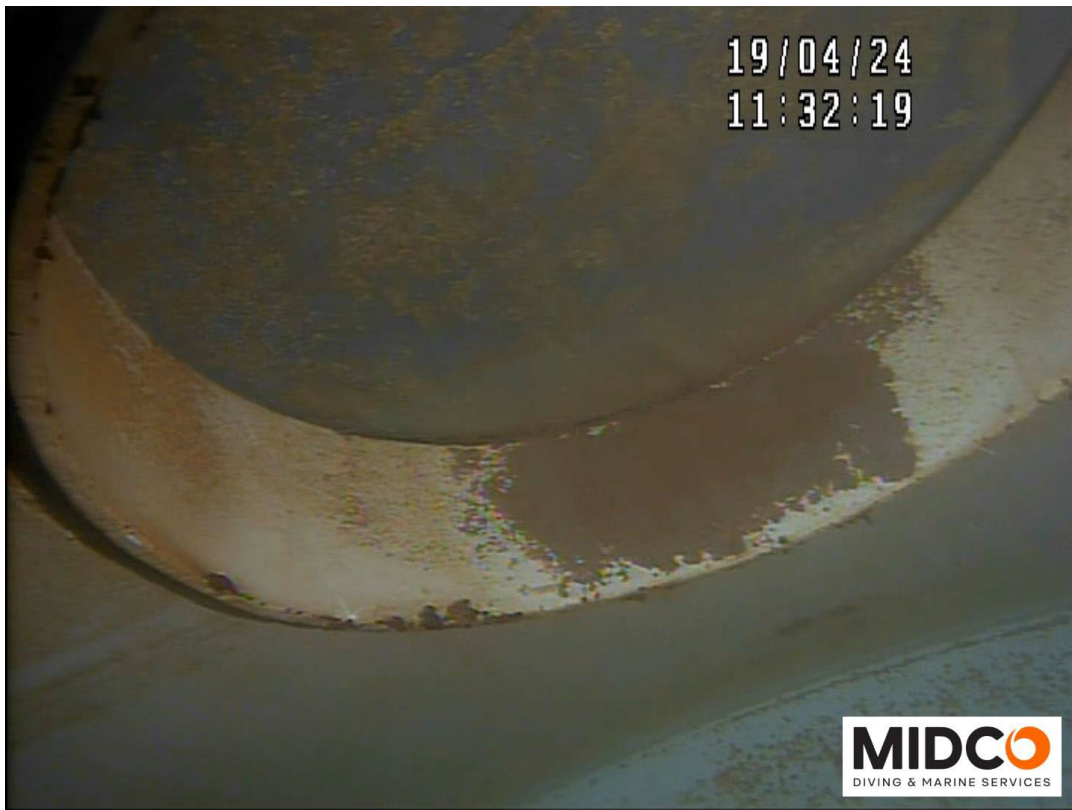
Man Entry #1 – Coating Failure with Corrosion Noted
