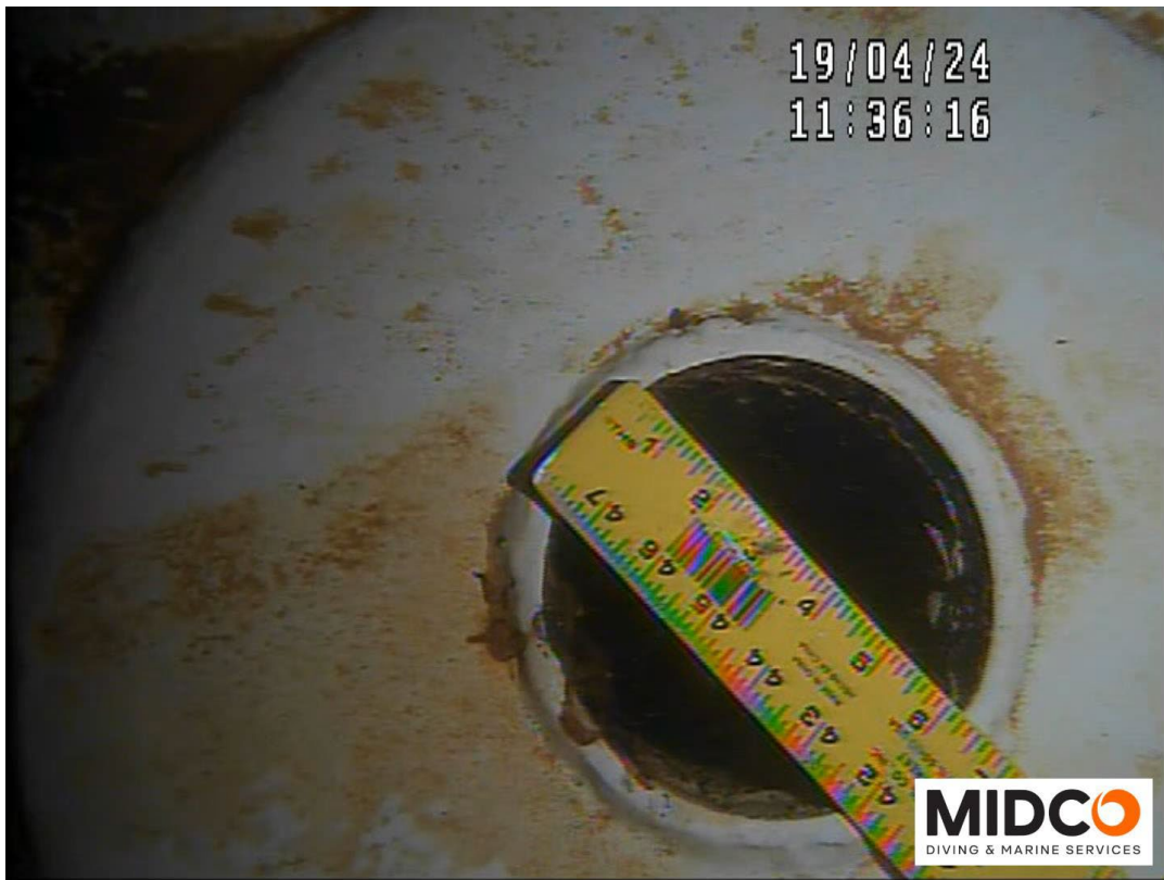
Drain Plumbing – Coating Failure with Corrosion Noted
