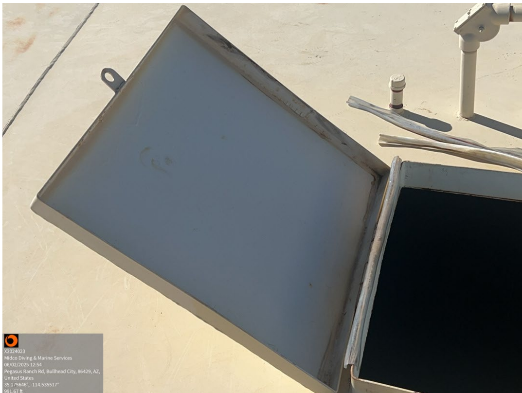
Access Hatch – Weather Stripping Deterioration Noted
