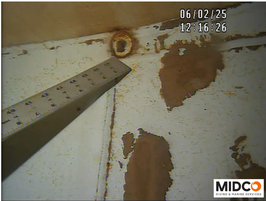
Floor to Wall Seam – Coating Failure with Corrosion & Pitting Noted
