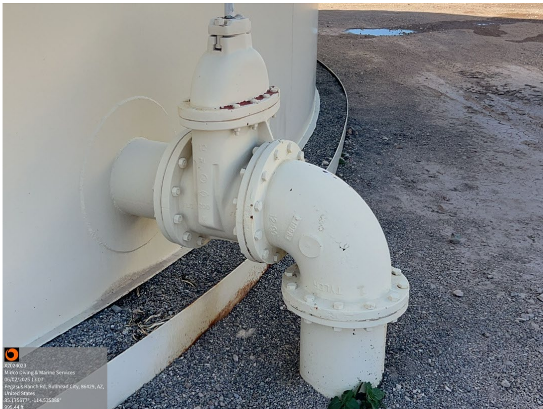
Inlet Plumbing – Coating Failure with Corrosion Noted
