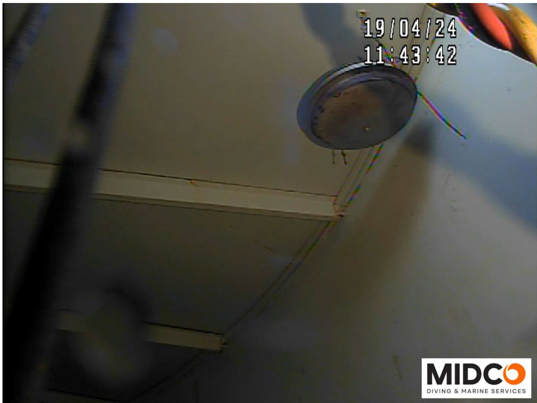
Manual Level Indicator Float – Non-Functioning
