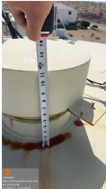
Roof Vent – Coating Failure with Corrosion Noted
