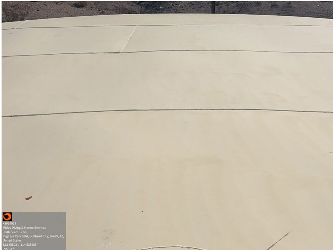
Reservoir Roof – Coating Failure Noted
