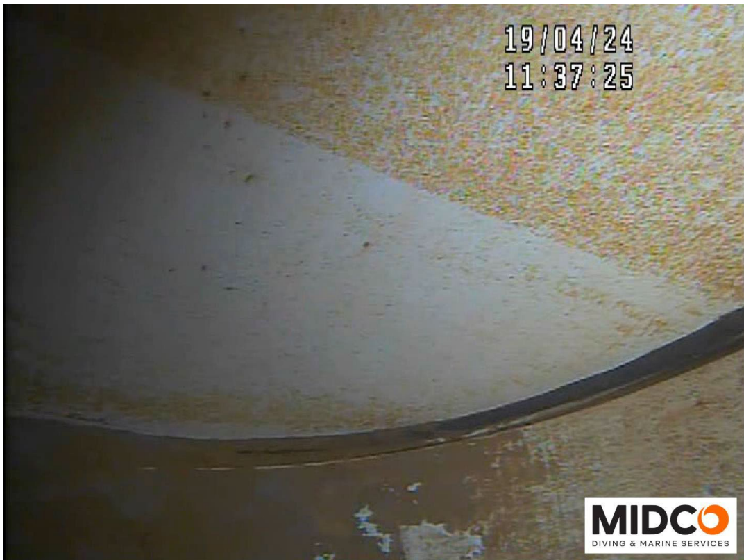
Man Entry #2 – Coating Failure with Corrosion Noted
